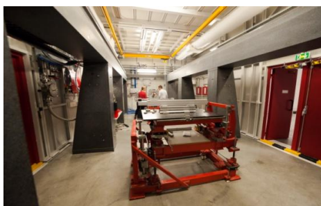
Figure 3. ID31 experimental hutch during construction of the beamline. Credit ESRF/P. Jayet.
