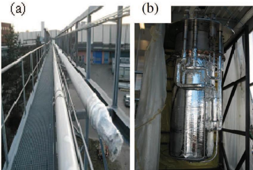
Figure 1. XATL1 cryogenic line under construction in April 2012 (a) and a view of one of the vertical cryostats during mounting of thermal insulation on the cryostat cold circuit and helium storage vessel (b).
